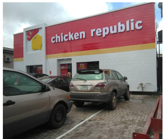
CMD Road, Magodo Lagos
