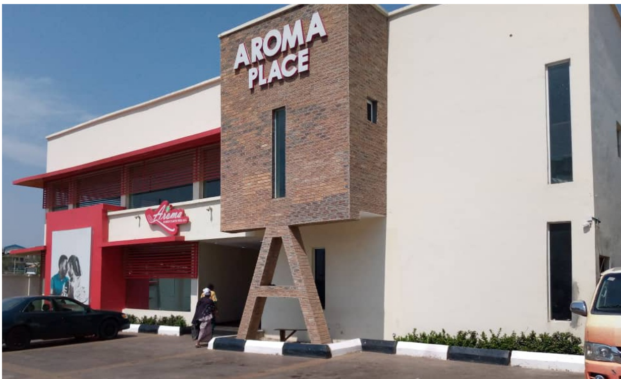
Unity Road, Ilorin, Kwara State
